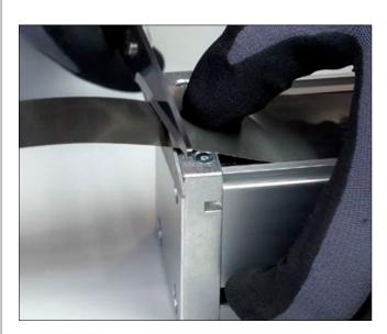
Fit the steel strip, which covers the spindle in the profile. This strip should be approximately 12 mm longer than the Support Profile.
